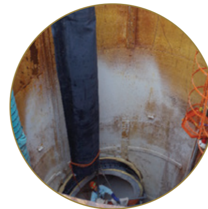
Inserting a folded pillow plug
