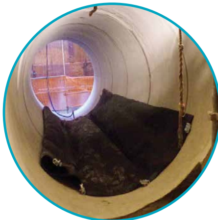
Placing – pillow plug should be positioned horizontally
