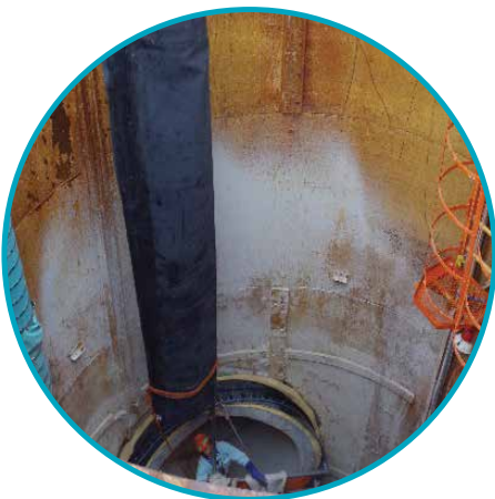
Inserting a folded pillow plug
