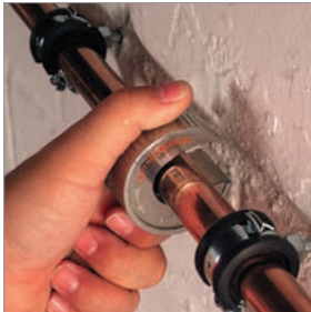
Pipe cutting possible near the wall
