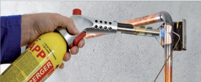
Brazing in gas installation
