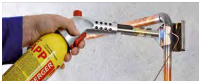
Brazing in gas installation
