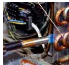
Brazing in refrigeration / air-conditioning technology
