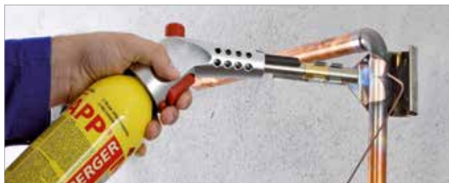
Brazing in gas installation
