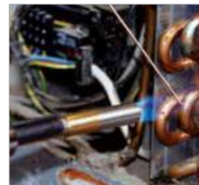
Brazing in refrigeration / air-conditioning technology
