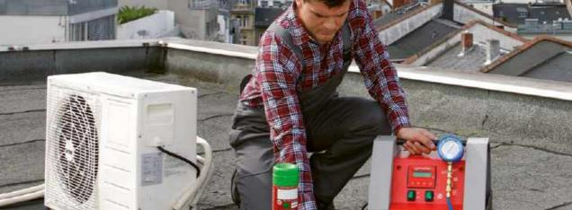
Set (No. 1000000138) includes: 2-stage vacuum pump, 2 low pressure gauges, 1 high pressure gauge R410A, 2 pressure hoses with ball valve à 2,500 mm, 2 bottle connection adaptors (1/4" SAE No. 173205, 5/16" SAE No. 173204), 2 reducing pieces 1/4" SAE F - 5/16" SAE M (No. 170016), precision digital scale up to 100 kg, automatic control, vacuum and pressure switch, mineral oil (No. 169200)
