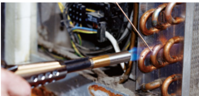
Brazing in refrigeration / air-conditioning technology
