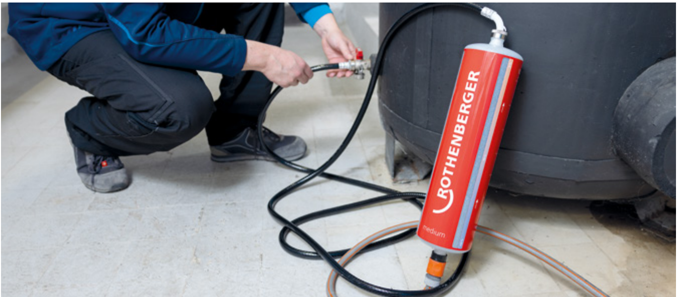
Filling heating systems according to standards
