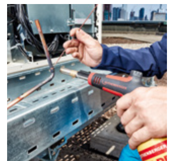
Brazing in refrigeration / air-conditioning technology
