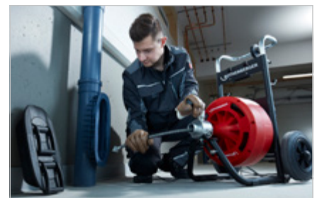
Cleaning of a down pipe with 16 mm spiral
